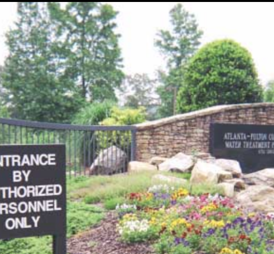
Atlanta-Fulton County Water Treatment Facility (Photo by VIDEX, Inc.)
