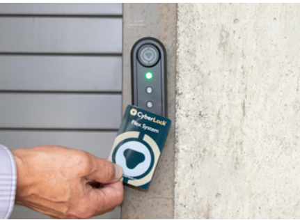
Using the FlashReader to access a hardwired door controlled by CyberLock Flex System
